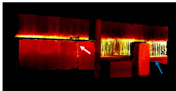
Figure 12. Textured 3D model obtained after the calculation of the rotation matrix and the translation vector for the 10 thermographic images needed to cover the wall. Temperatures rise from 24.5°C (dark red) to 31.5°C (white).
